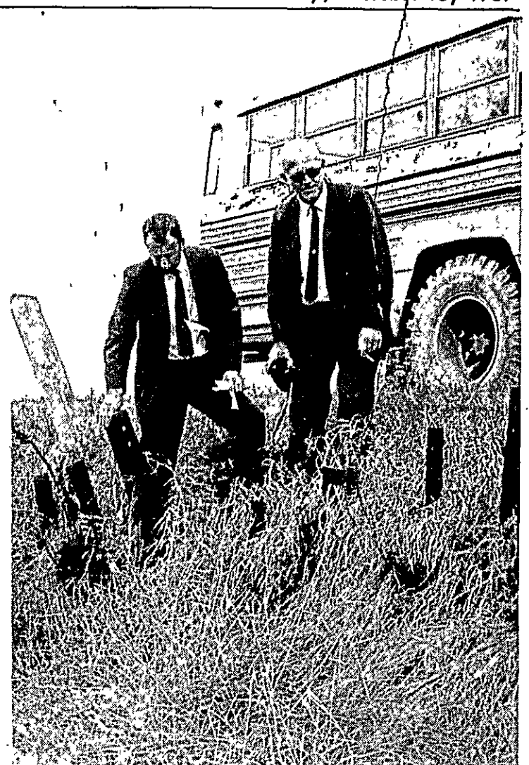
County Road Commission Engineer-Manager, Don Haske, on left, and Commission Chairman Paul Nobis examine area along roadway where crews have buried discarded grader blades to inhibit erosion of road shoulders and ditch banks. Several roads in the county with similar conditions are among those scheduled for reconstruction to provide greater safety and sounder roadbeds.
