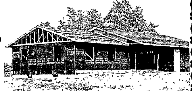
1013 E. CASS STREET--NOW UNDER CONSTRUCTION
