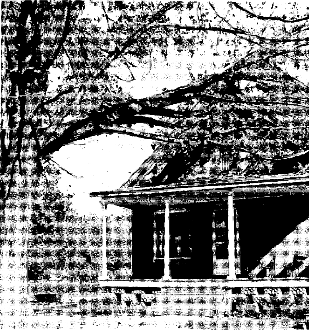
HIGH WINDS TOPPLE LIMB ON HOUSE
