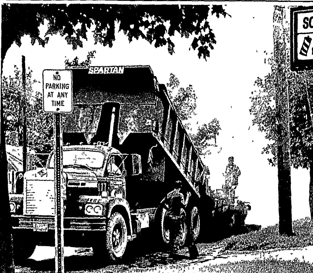
Getting in some road-repair and repaving work before the snow-flies this year, the workmen put the finishing touches on a paving project along M 21 at Traver Street in St. Johns.
