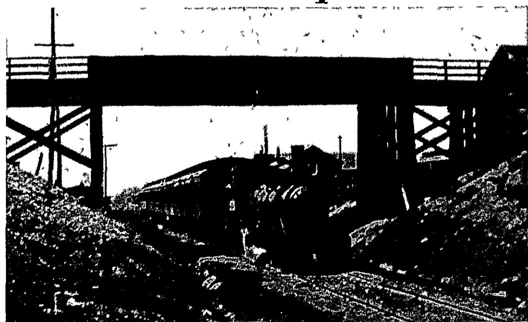
WHITTEMORE STREET BRIDGE OVER THE GRAND TRUNK
