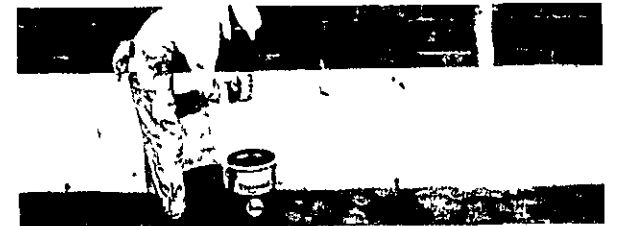
BRUSH ON a heavy coat of THOROSEAL up about 2'4" on walls. For extra protection where water pressure is heaviest Dampen area first. Then apply a full base coat of THOROSEAL to entire wall, beginning at the top.
