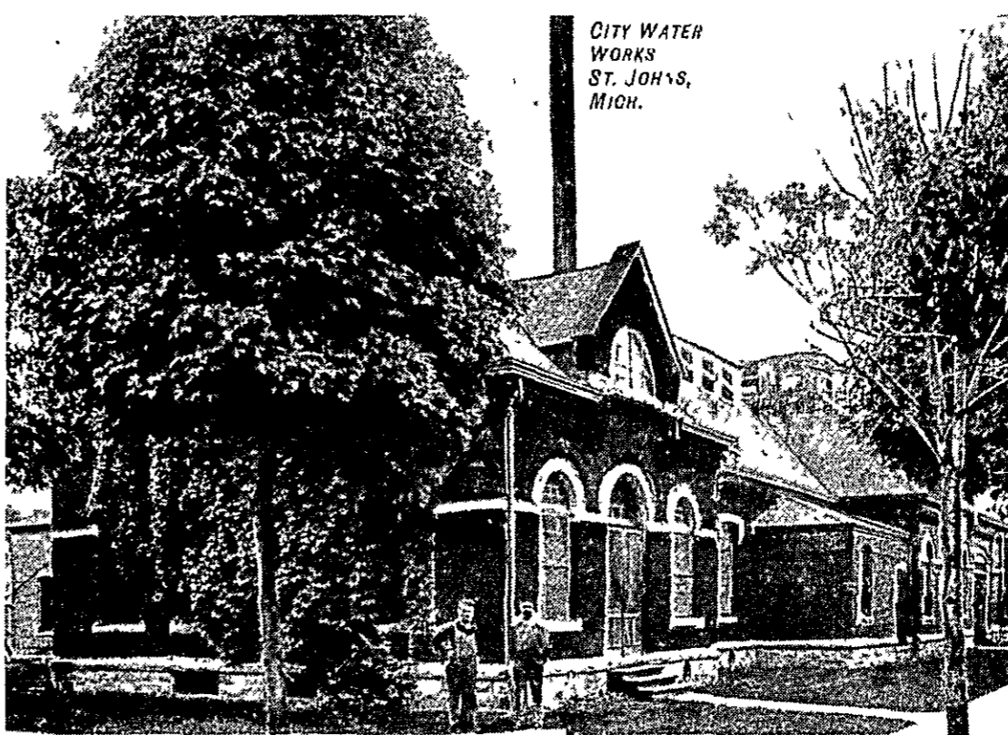
OLD ST. JOHNS WATER PLANT ON CITY'S NORTH SIDE
