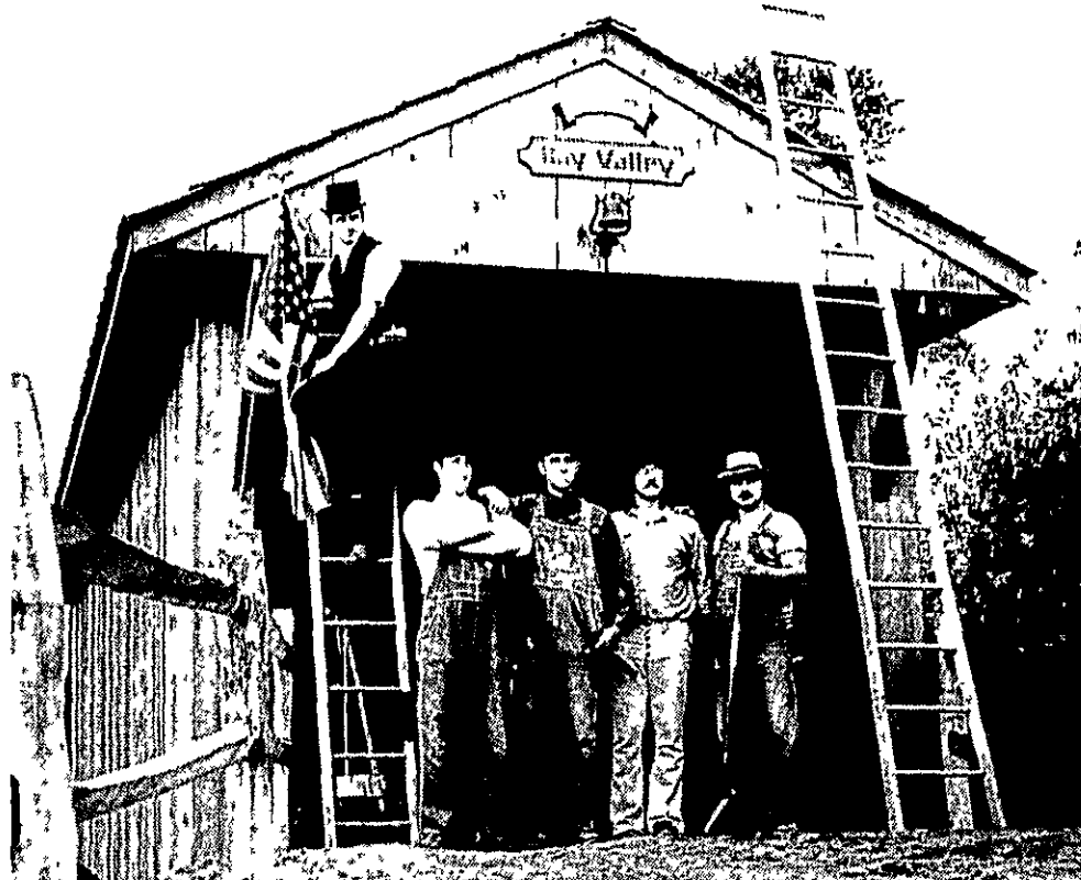
WORKERS COMPLETE COVERED BRIDGE
