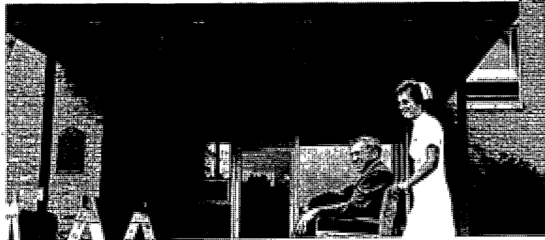
What's it like to be a patient at Clinton Memorial Hospital? Central National Bank President Harold Wellman gets a tour with Mrs. Pat Simmet, RN, director of nurses. Arriving at the hospital at 805 S. Oakland, Wellman gets a look at construction of a third floor to the Fehling addition.
