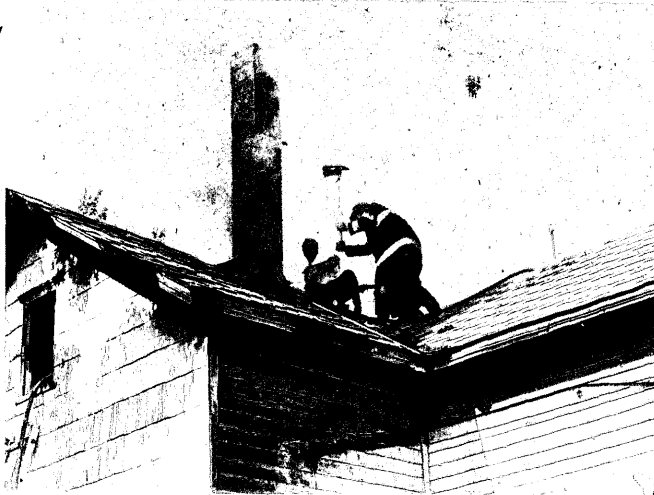
St Johns firemen, assisted by DeWitt firemen, battle a house fire Tuesday on Yallup Road near DeWitt. The fire in the house, owned by Lyle Hallead, is believed to have been caused by an electrical malfunction.
