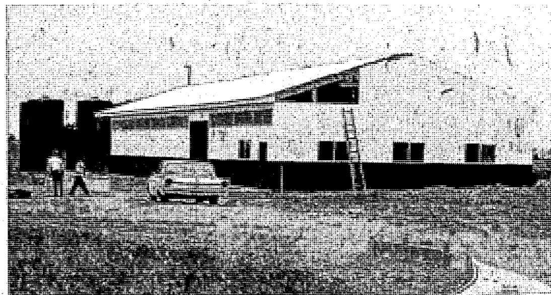
NEW FARMERS PETROLEUM BUILDING
