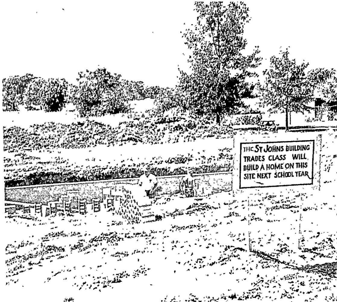
Building trades class of St. Johns High School will be building a house on this site on Lansing Street. Helping the boys get started are masonry contractor, Richard (Sonny) Cornwell, left, and his son, Richard.
