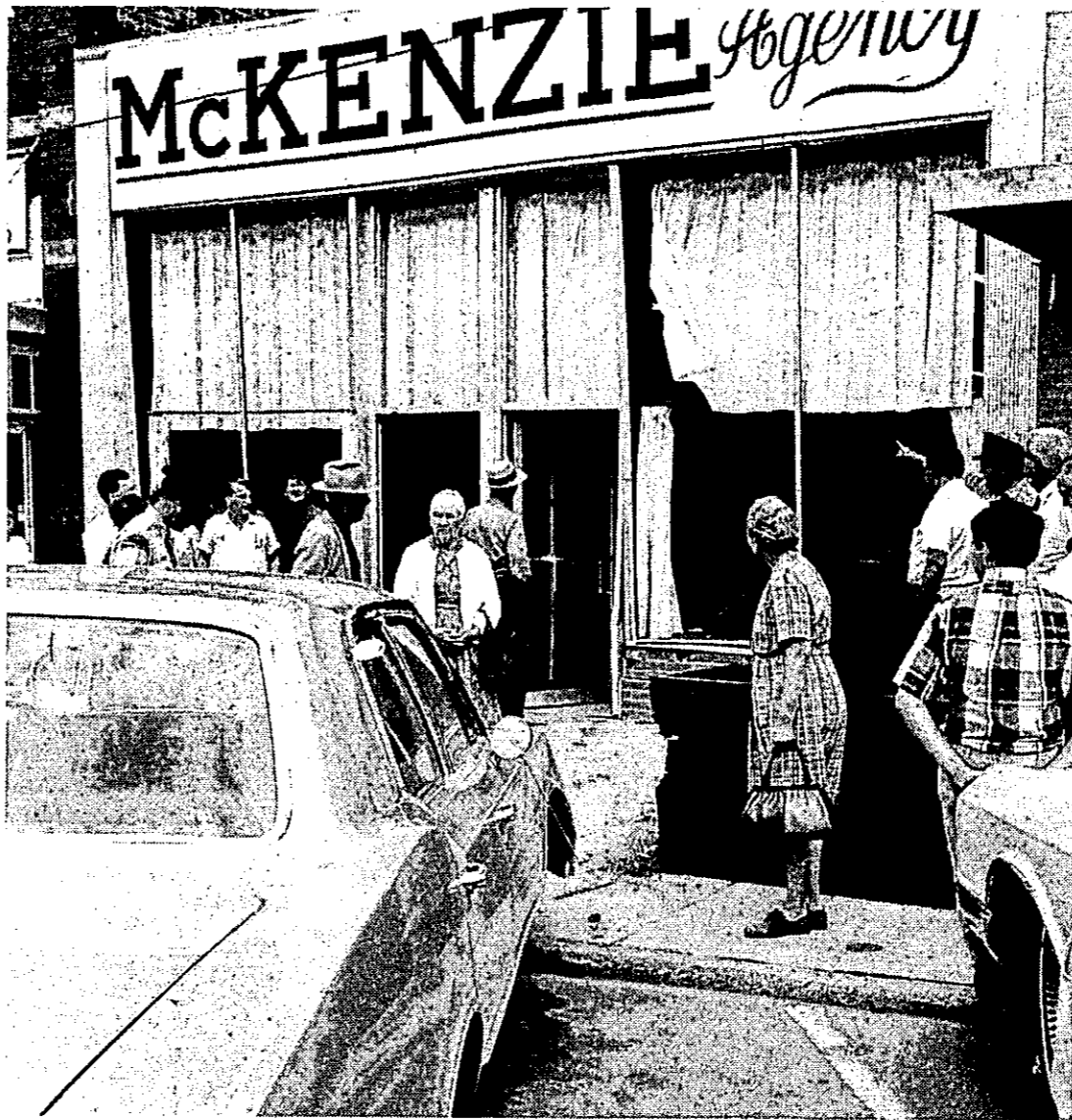
Car smashes front of downtown building
