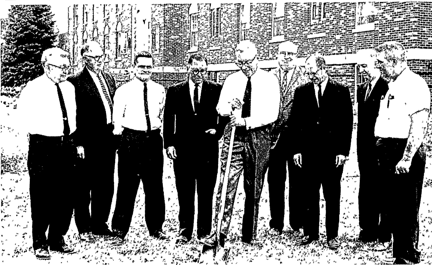
Hospital officials break ground for addition
