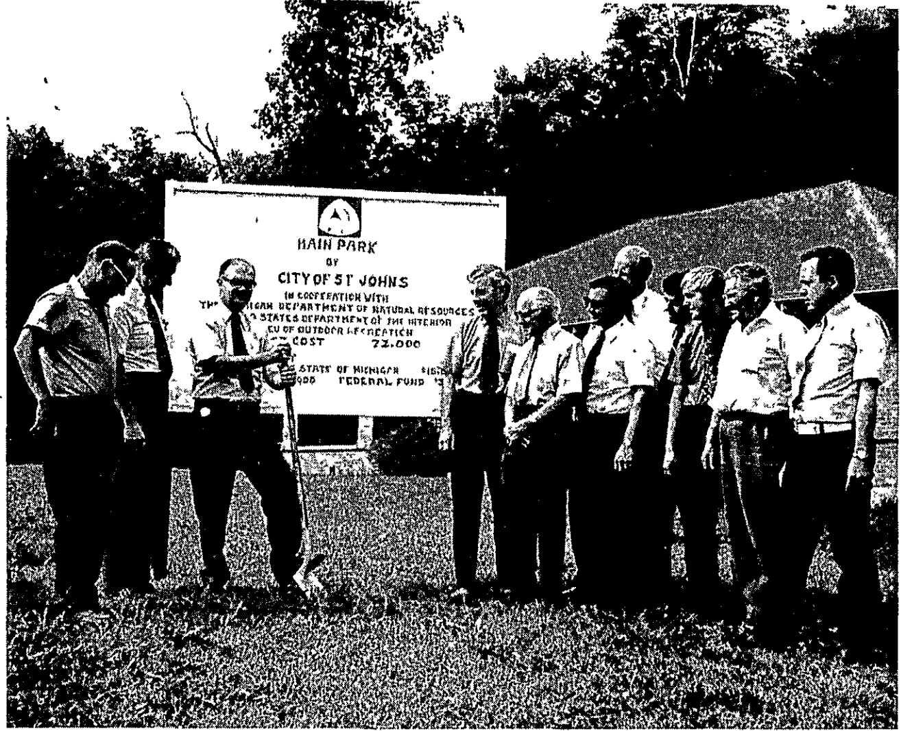
Break ground on park project
