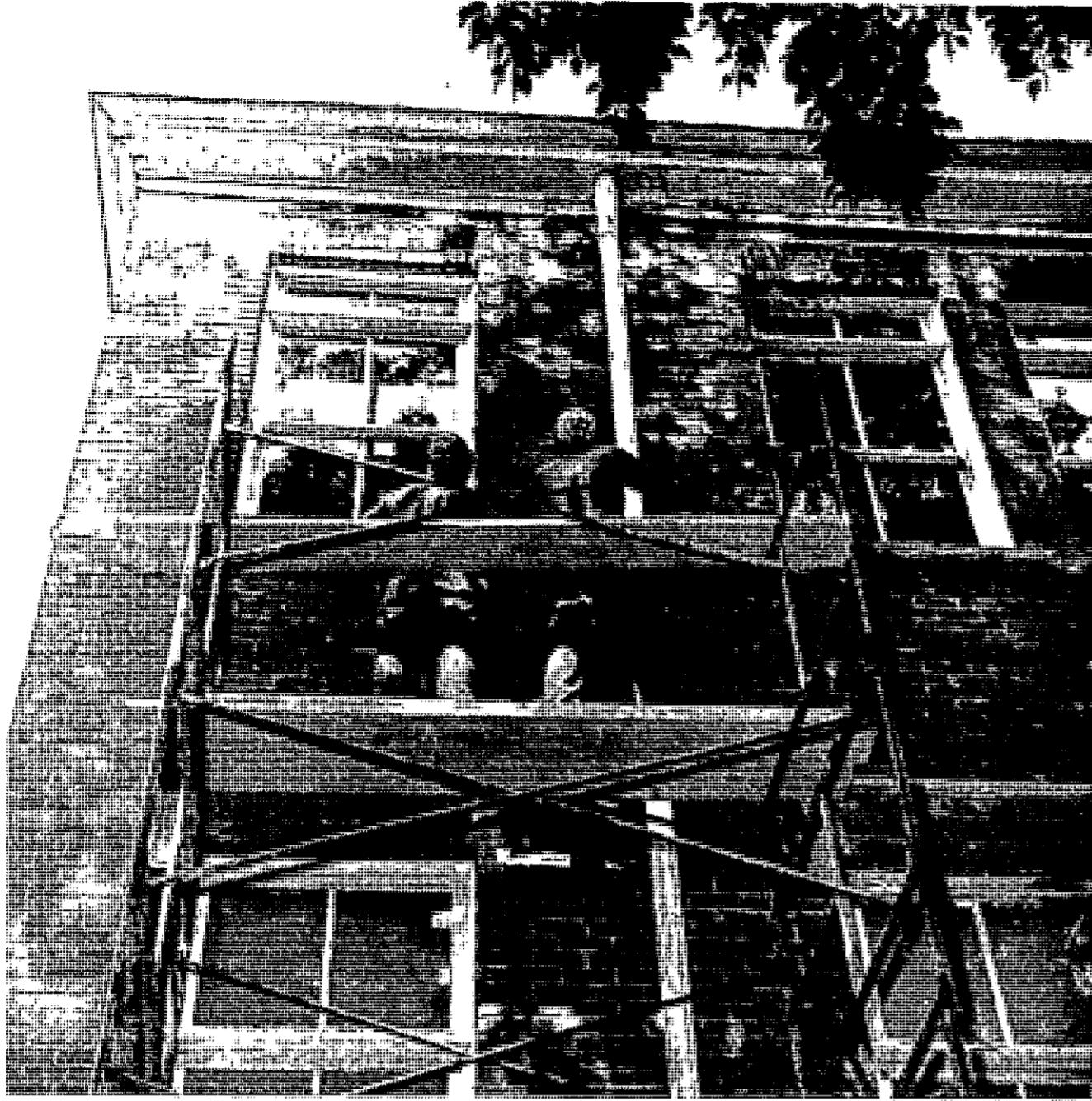
Repairs are underway at Central School as Richard Cornwell and Terry Adams proceed with the task of facing up loose or missing brick work on the building.
