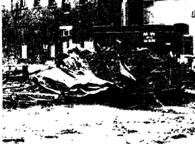
Fire destroyed this building behind the downtown business section of Ovid and, up to a week later, smoke was still curling from the debris.
