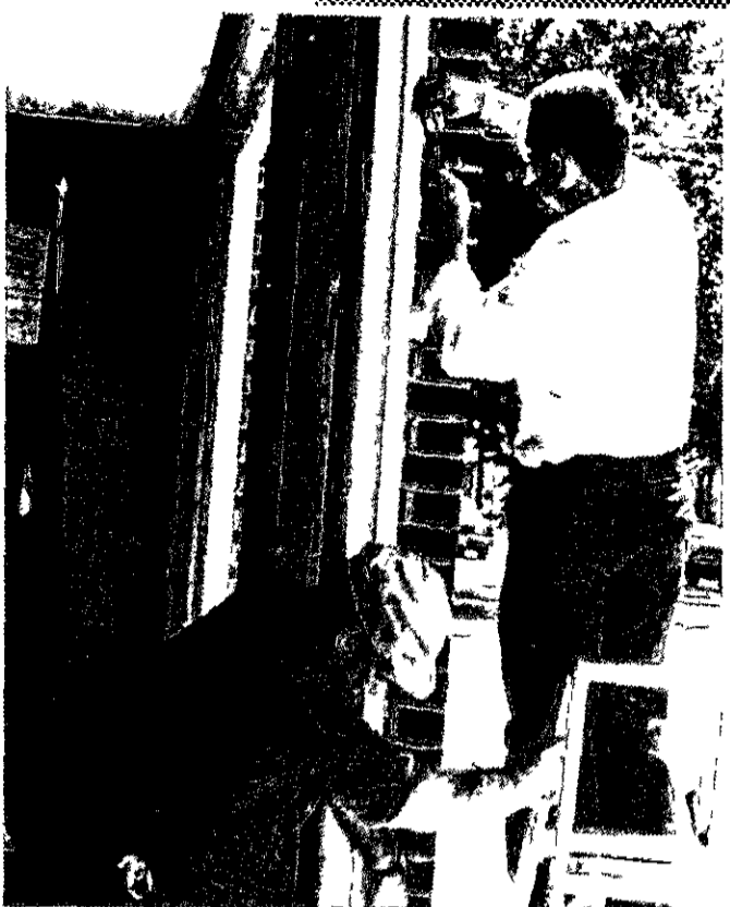
It was an open air office for a while in Ovid Village Hall while new windows were being installed. It's not the only new look in town—streets are being repaired and business buildings are getting fresh coats of paint.
