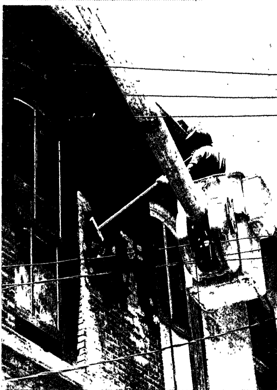
Mike Taylor gets an assist from a boom truck while repairing and painting store fronts in Ovid. The Ovid Businessmen's Association prompted the move to have the village's downtown area provided with a new look with individual cooperation from store owners.
