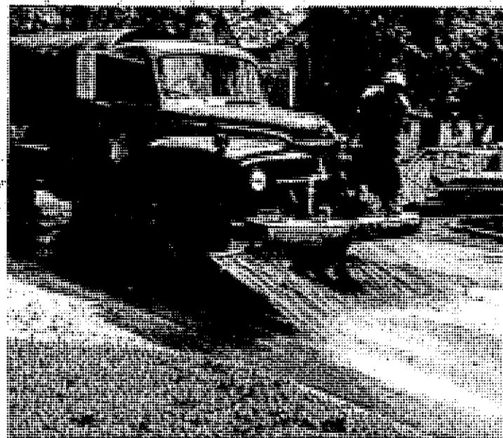
OLD FIRE TRUCK WITH A NEW JOB
