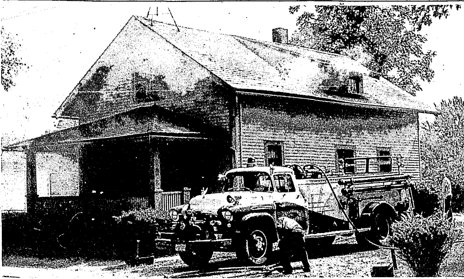
CLINTON AVENUE FIRE
