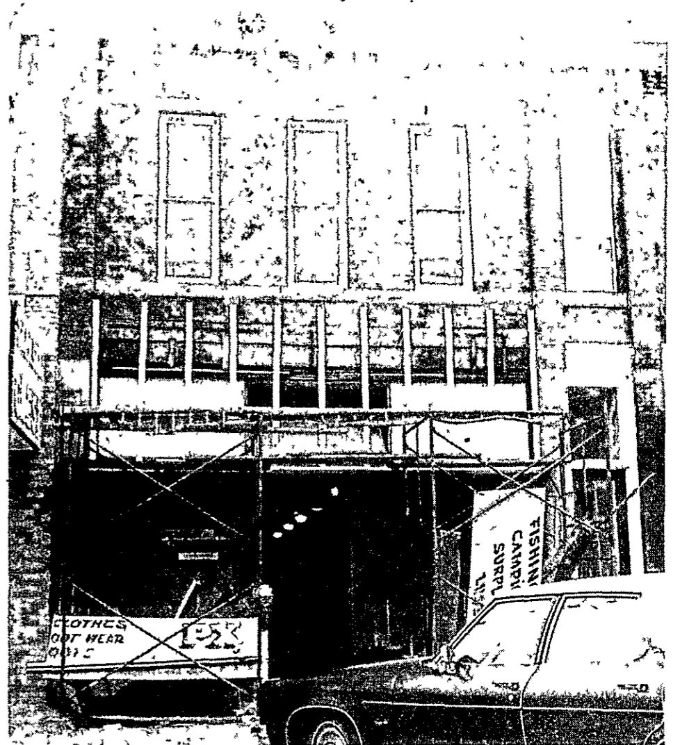
Another business to get a new look in St. Johns is the PX Store. Remodeling is currently underway on the front of the store owned by Jack Andrews.
