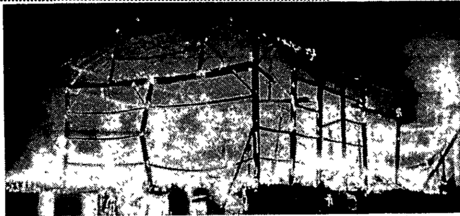
Fire destroyed this barn on Rabbit in Ovid last week and the Shlawassee County Sheriff's Dept reports arson is suspected and the incident is under investigation. The barn, owned by an Ovid Church, was not in use at the time of the fire.
