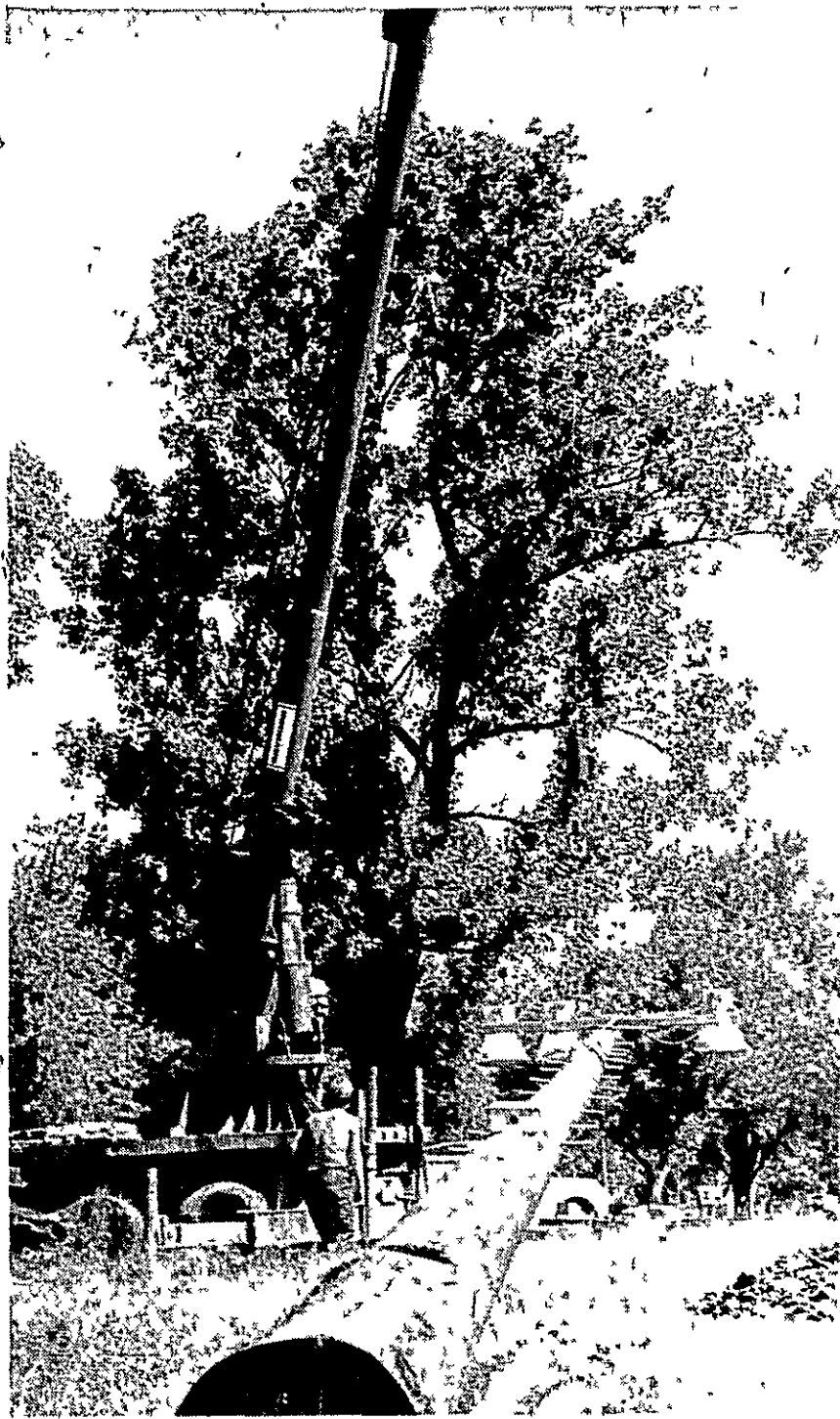
Contractors install new lights on the Fowler Little League field. Following the erecting of lights on the Fowler field, contractors will begin work in St Johns, where Little League teams will also be playing under the lights.
