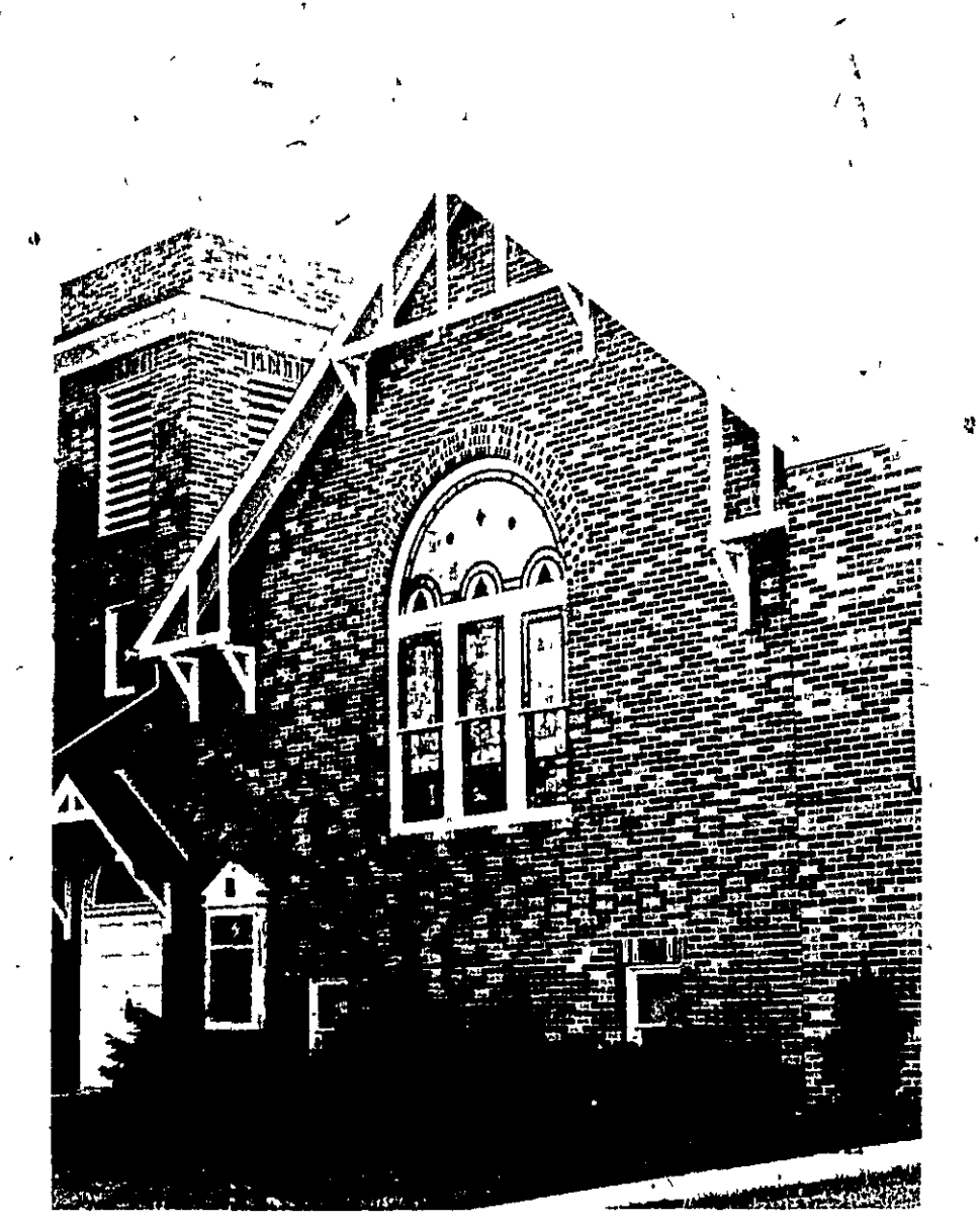
DeWitt United Methodist Church N Bridge St.
