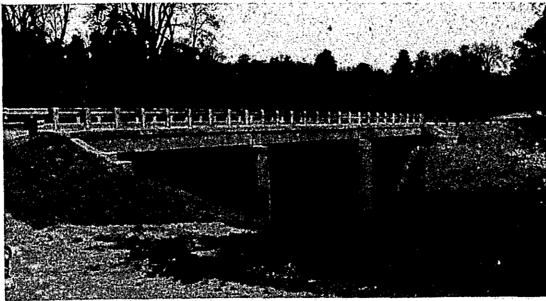
Final touchup work done on new bridge
