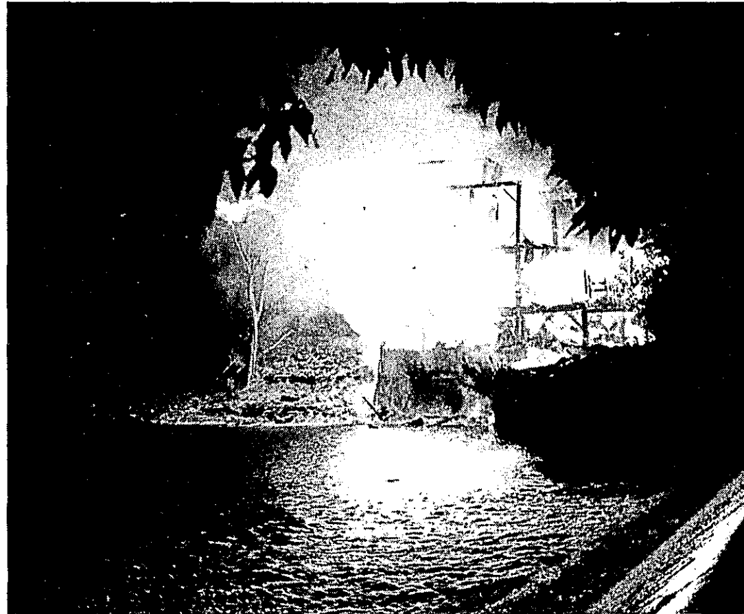
Roaring flames that are killing the 135-year-old grain elevator at Elsie created this ironically picturesque scene from the north side of the Maple River immediately adjacent to the Elsie dam. Elsie firemen had no chance to save the old structure.
