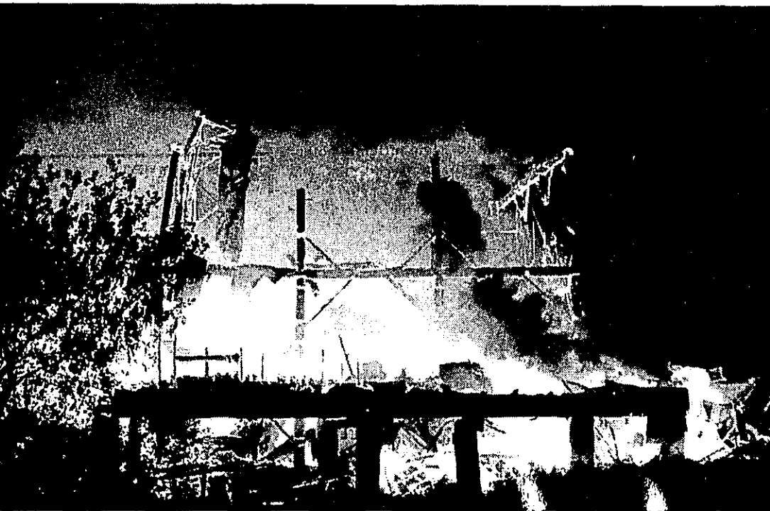
Like a glowing skeleton, flaming framework of the Ovid Farmers Elevator at Elsie stands starkly against a dark early-morning sky Thursday minutes before much of it crumbled. The fire, which started about 3:40 a.m., destroyed the landmark, over 135 years old, which stood along the Maple River.
