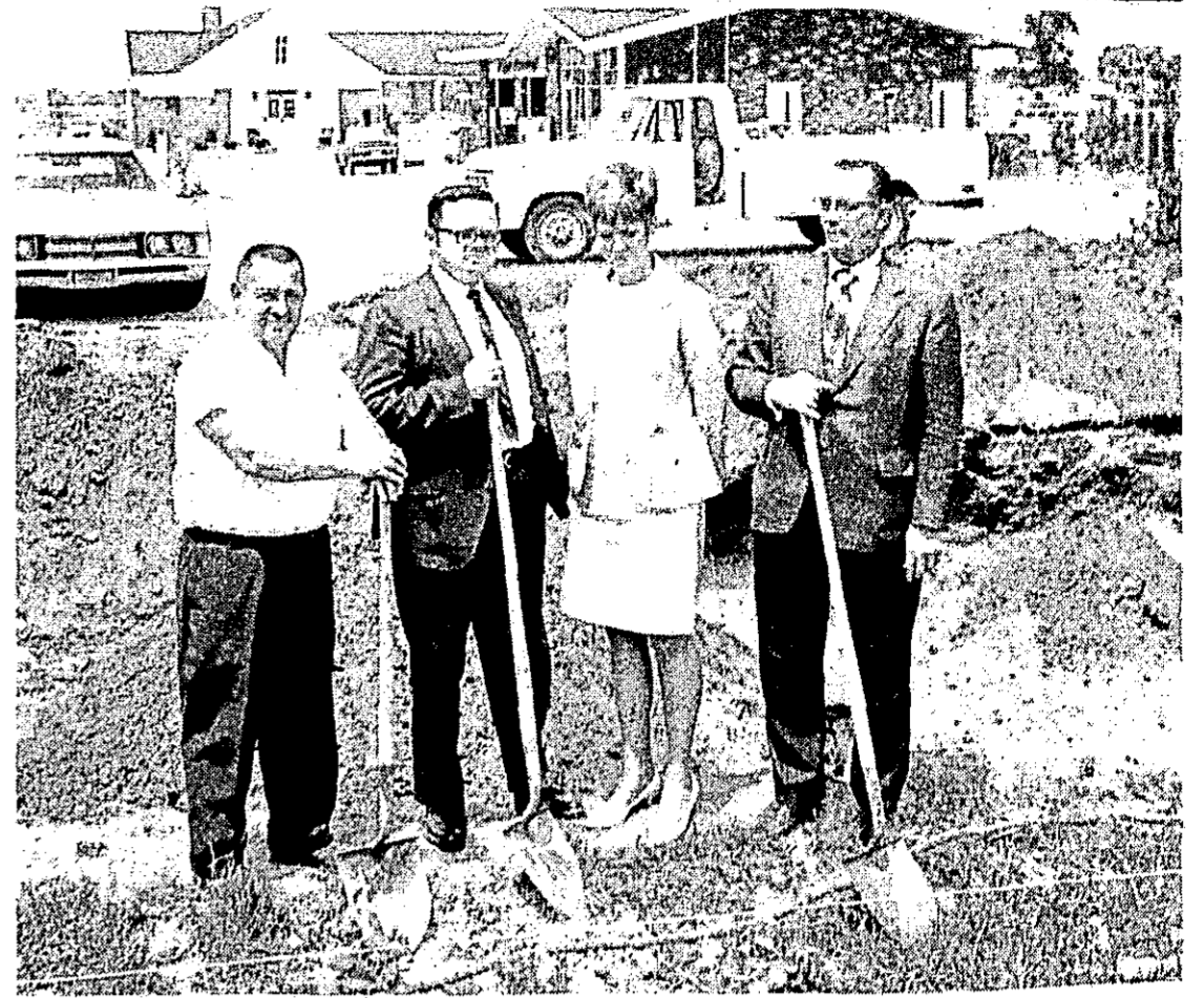
DeWITT PROJECT UNDERWAY
