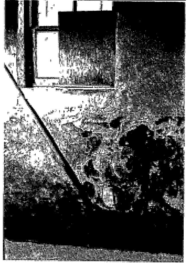
This wall at Central School requiring refinishing and broken window replaced.
