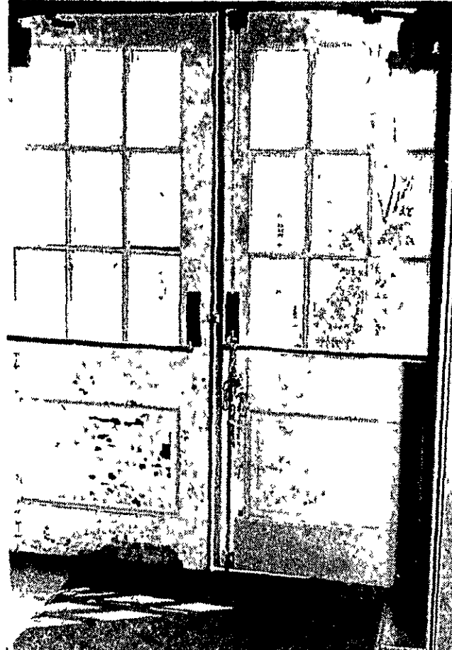
An interior view of a door at Rodney B. Wilson Junior High shows the need for repairs.
