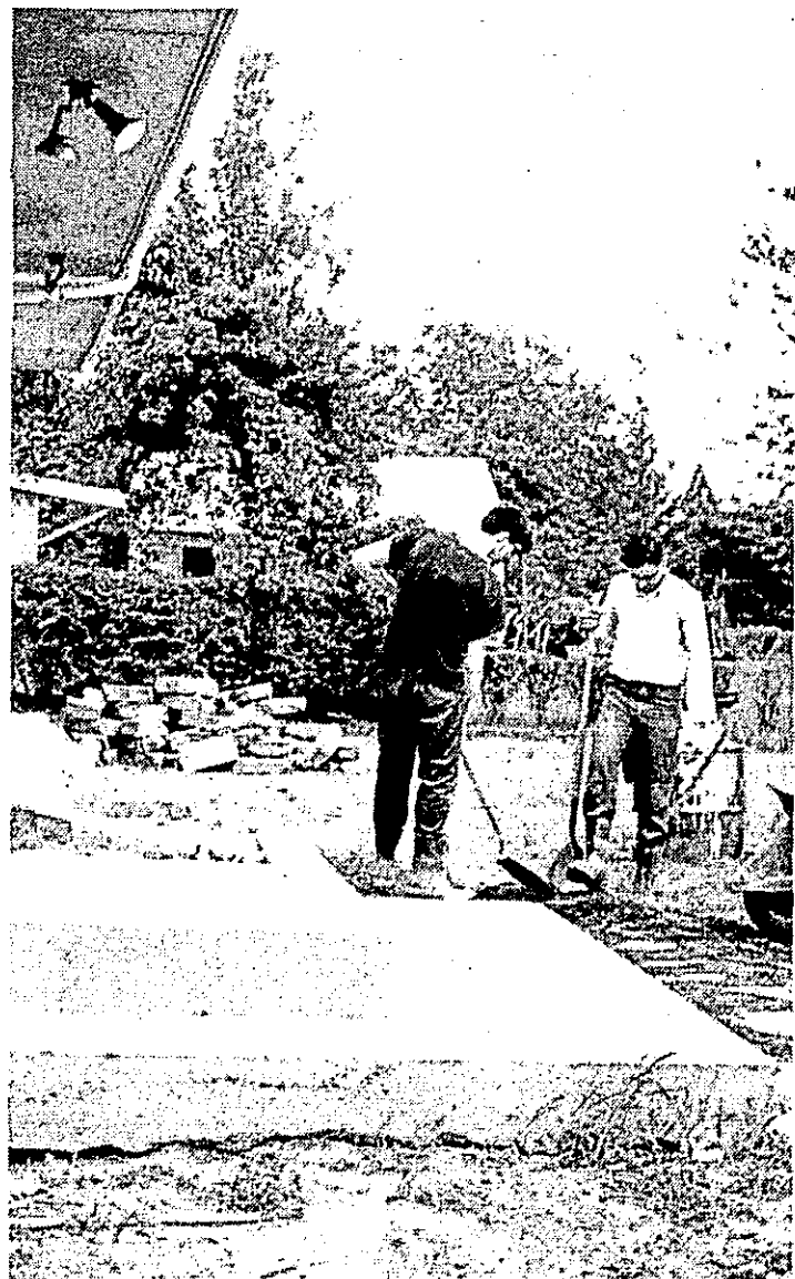
Building a patio.
