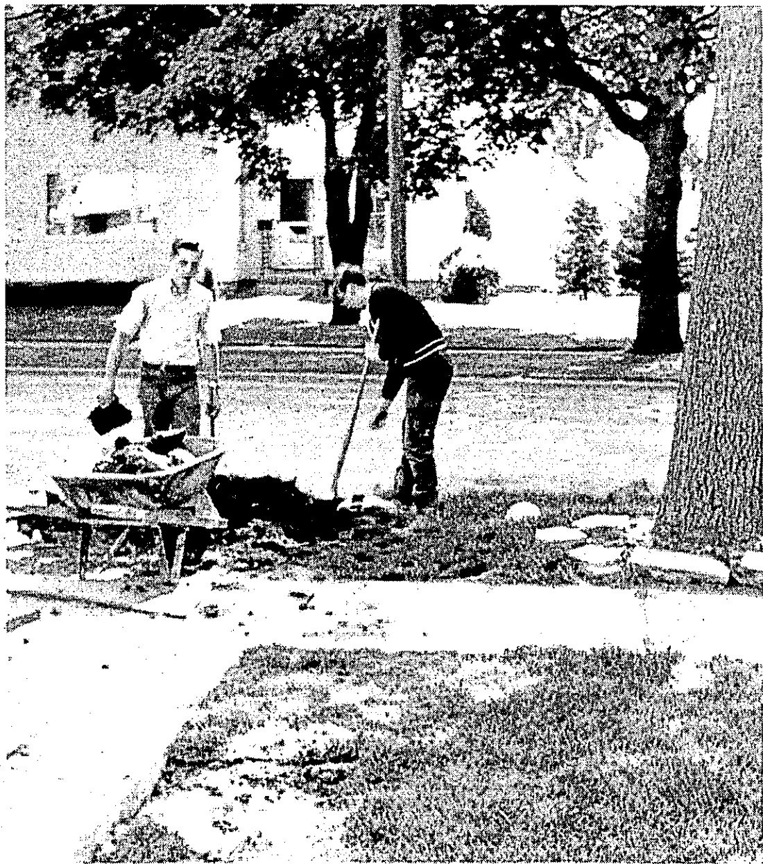
Putting in a driveway.
