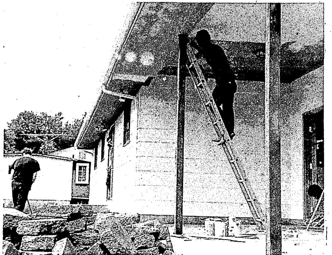
Finishing touches on the porch.
