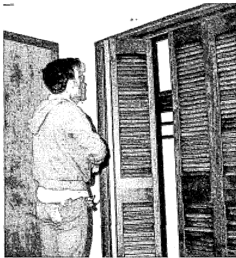
Ed Harr touches up the window frame as one of the final jobs on the exterior of the house.
