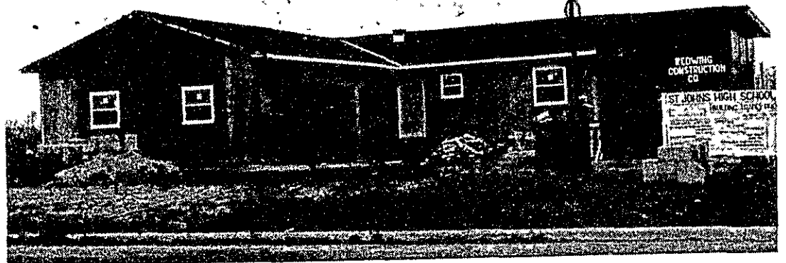
REDWING CONSTRUCTION CO.
