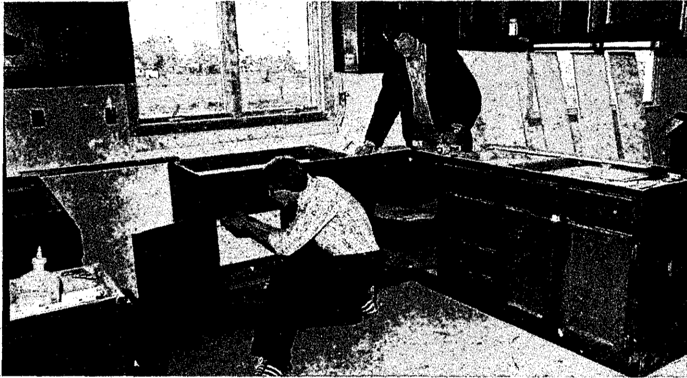
Workers install kitchen cupboards.
