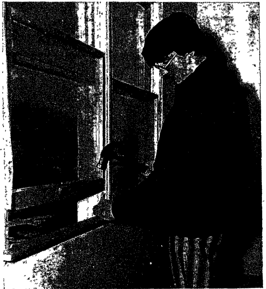
St. Johns student sinks nails in sash encasing Anderson windows.
