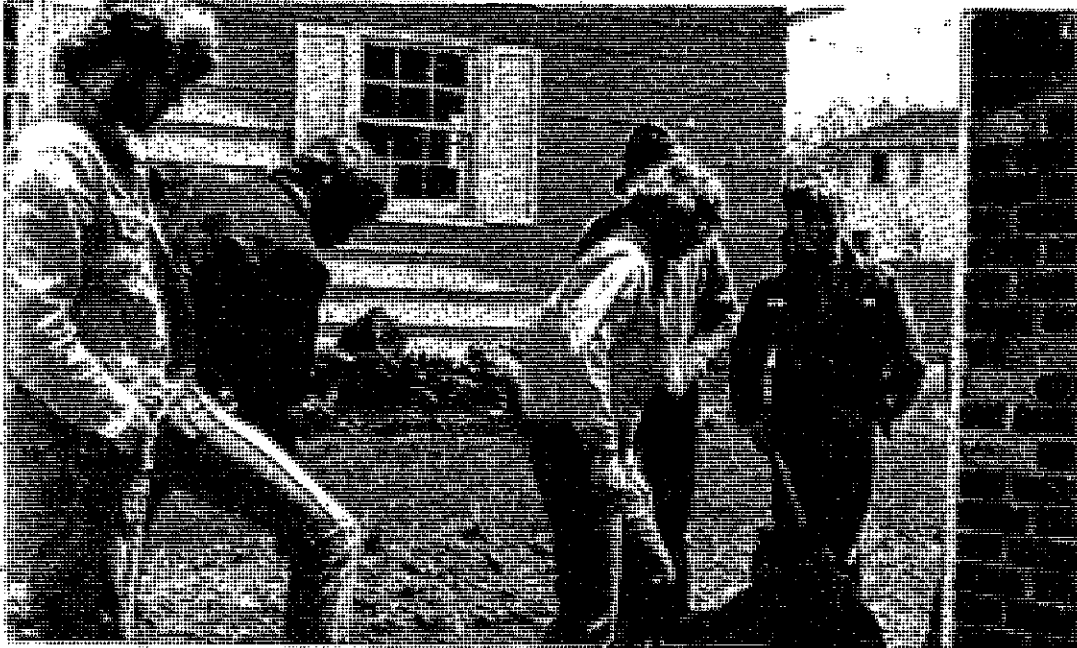
Getting ready to pour cement are instructor Bob Niemi and his building trades class.
