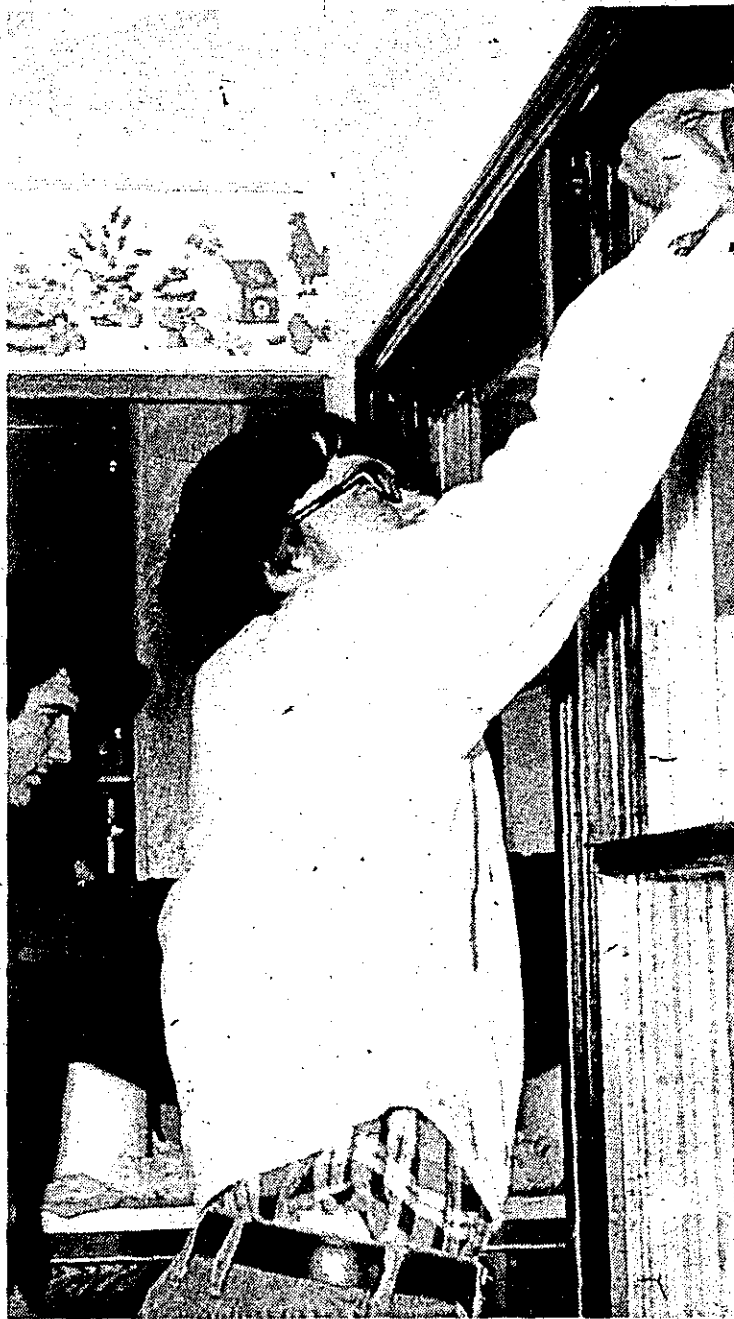
Larry Wirth (left) and Carl Huhr make sure the windows seal properly.
