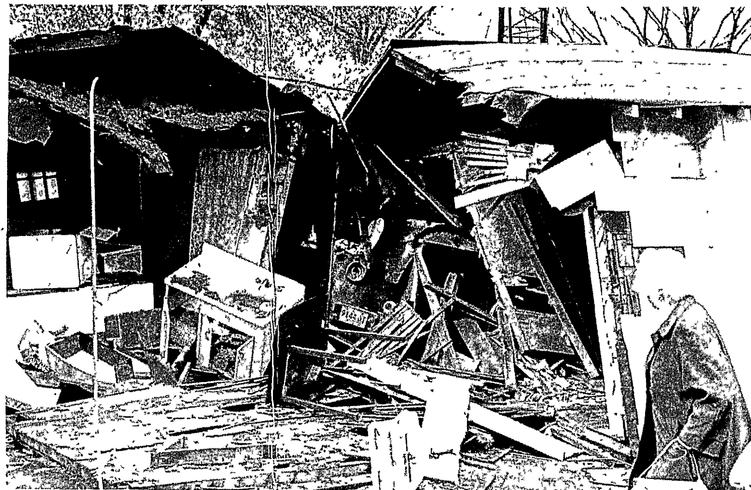
It looks like a tornado hit, but actually this house near the corner of State Road and US-27 was blasted apart by a tanker
