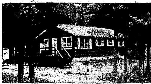
ORIN ARGENSINGER CONDENSARY ROAD
