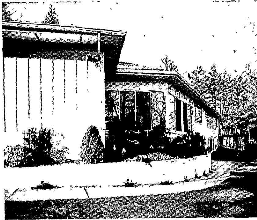
Prefinished panel siding is not only functional, it's also attractive. Exterior of this luxury home is covered with Colorlok panel siding, a product of Masonite Corporation. Unique 2-piece battens, comprised of a hardboard backer strip and color-matched aluminum cover, conceal nailing and serve to cover the joints. Prefinished soffit system is compatible with the exterior hardboard siding.
