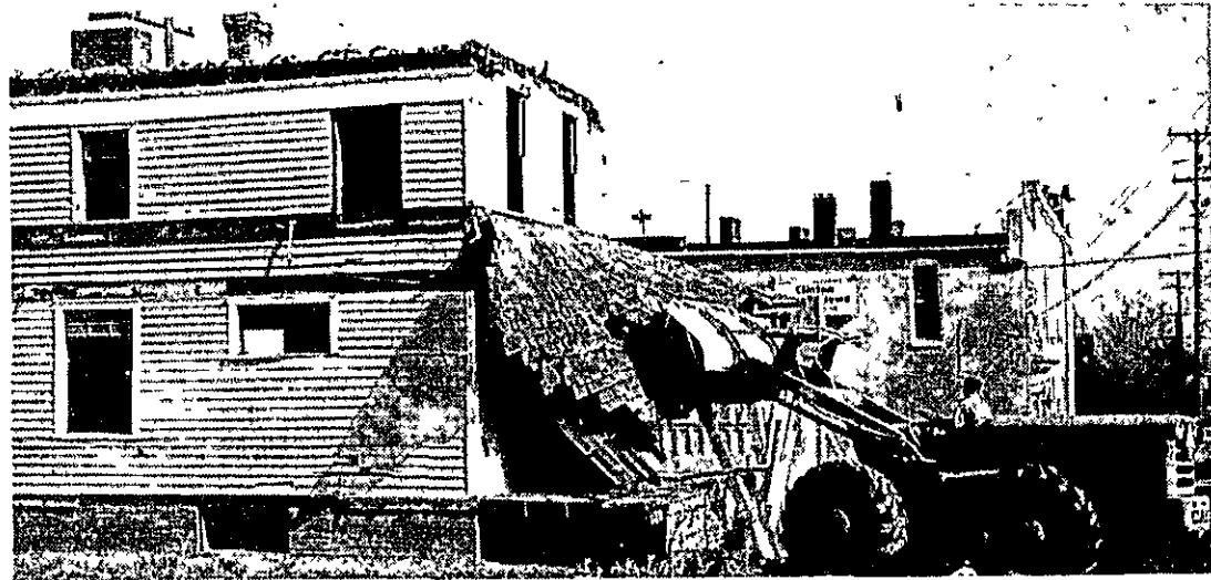
Jack Smit, president of Northwest Salvage Incorporated of Williamston and several employees have been busy this past week with the tearing down of a house at 105 Spring Street. Smit, estimates the age of the structure at 60 years and says it was unusual in that most of the wood used in its construction was oak and maple, (the majority of homes built at that time were pine).
