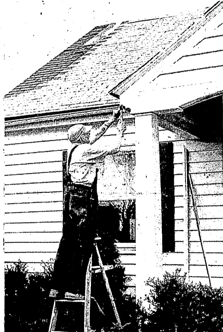
FWOYLER'S ED McCLOY AT WORK . . . new roof, porch work done
