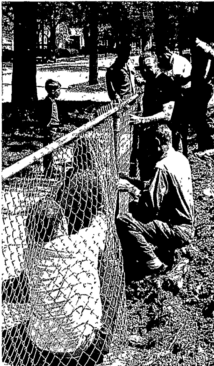
PLAYGROUND PROGRESS MADE
