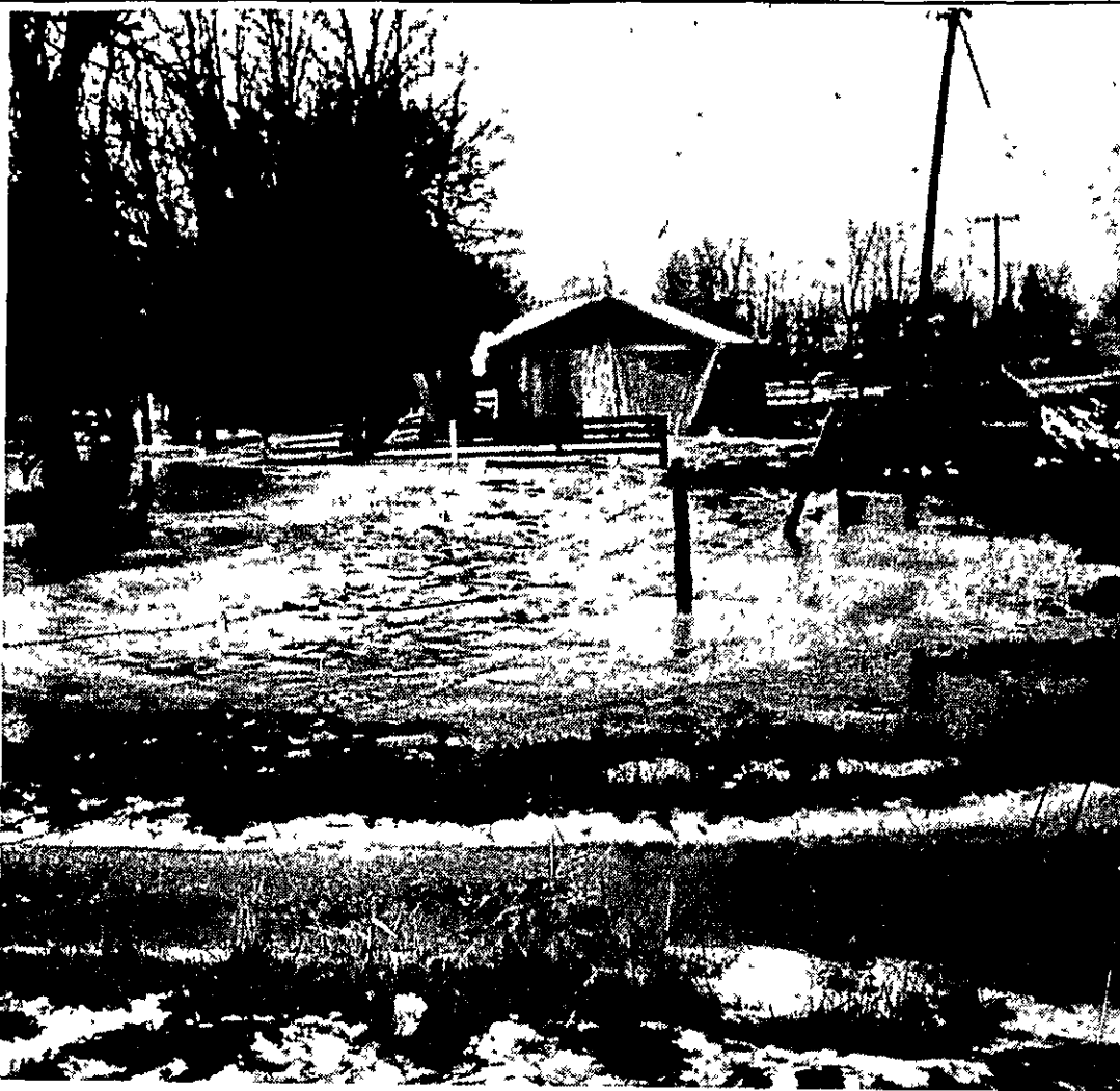
Buildings constructed in the floodplain of a river are often made use-less in times of high water. This building was built along the Looking Glass River west of DeWitt.
