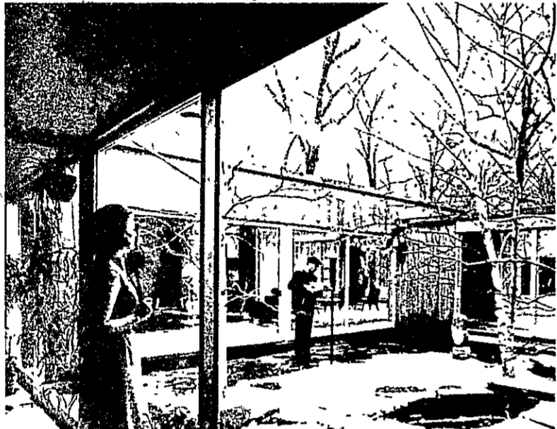
THE ROMAN-STYLE ATRIUM, an open-air courtyard built inside a home, is becoming increasingly popular for residences on small lots or in crowded neighborhoods. Living space is oriented inward to private natural beauty tailored to the owners' taste. Window walls of Thermopane insulating glass enable the interior courtyard to be enjoyed whether indoors or outdoors. A refreshing view is provided, no matter what the season.
