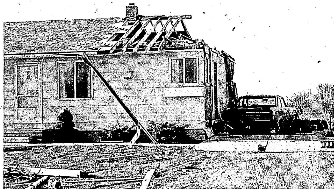
GARAGE DISAPPEARED IN STORM
