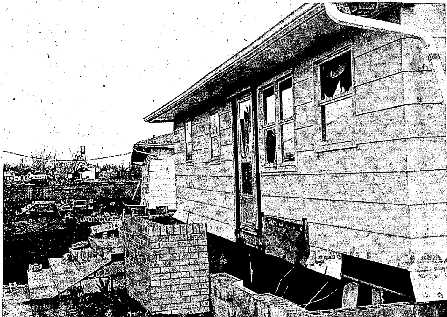
HOMES MOVED OFF FOUNDATION BY TORNADO'S FORCE
