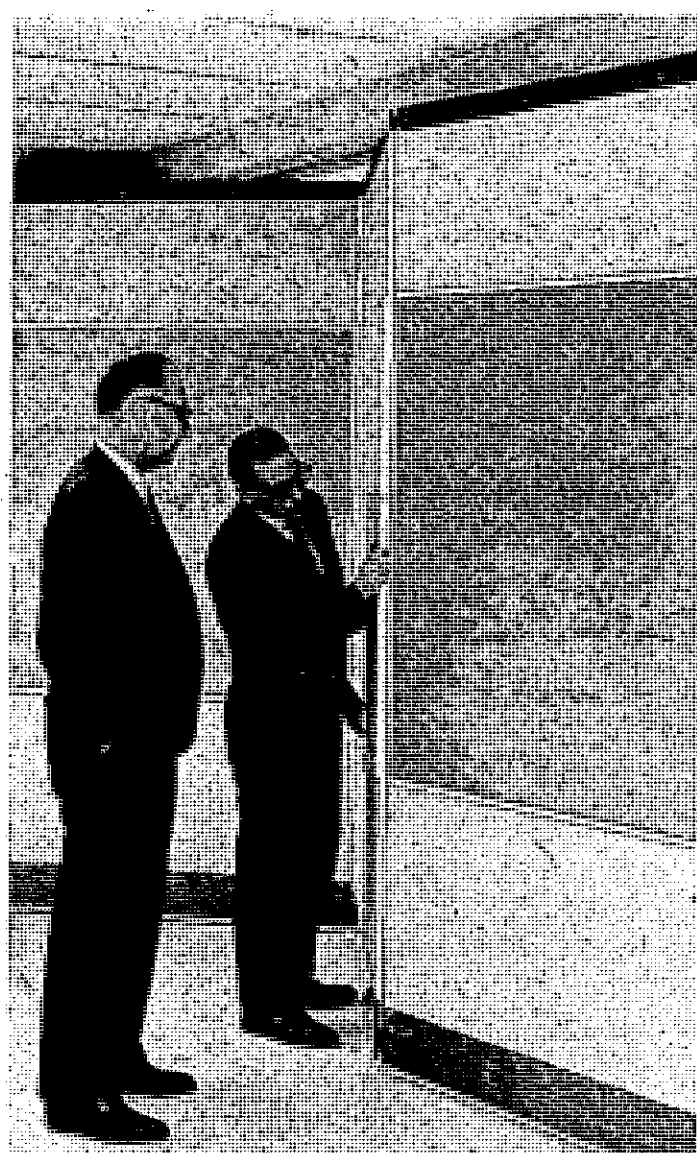
St. Johns Public Schools Administrative Assistants Walter Nickel and Steve Bakita inspect the seal between two sections of a folding partition between two classrooms at Riley Elementary School. The partition, when locked in place, makes the room as sound-proof as a concrete block wall would.
