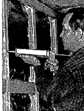
WOOD BEAM EFFECT CAN BE ACHIEVED in remodeling projects through "Vinylfold," vinyl-surfaced hardboard that folds into the shape of a beam. Complementary to wall paneling, the beams come in lengths of 12, 14 and 16 feet. Apply to ceilings of plaster, drywall or ceiling tile by nailing to furring strips.
