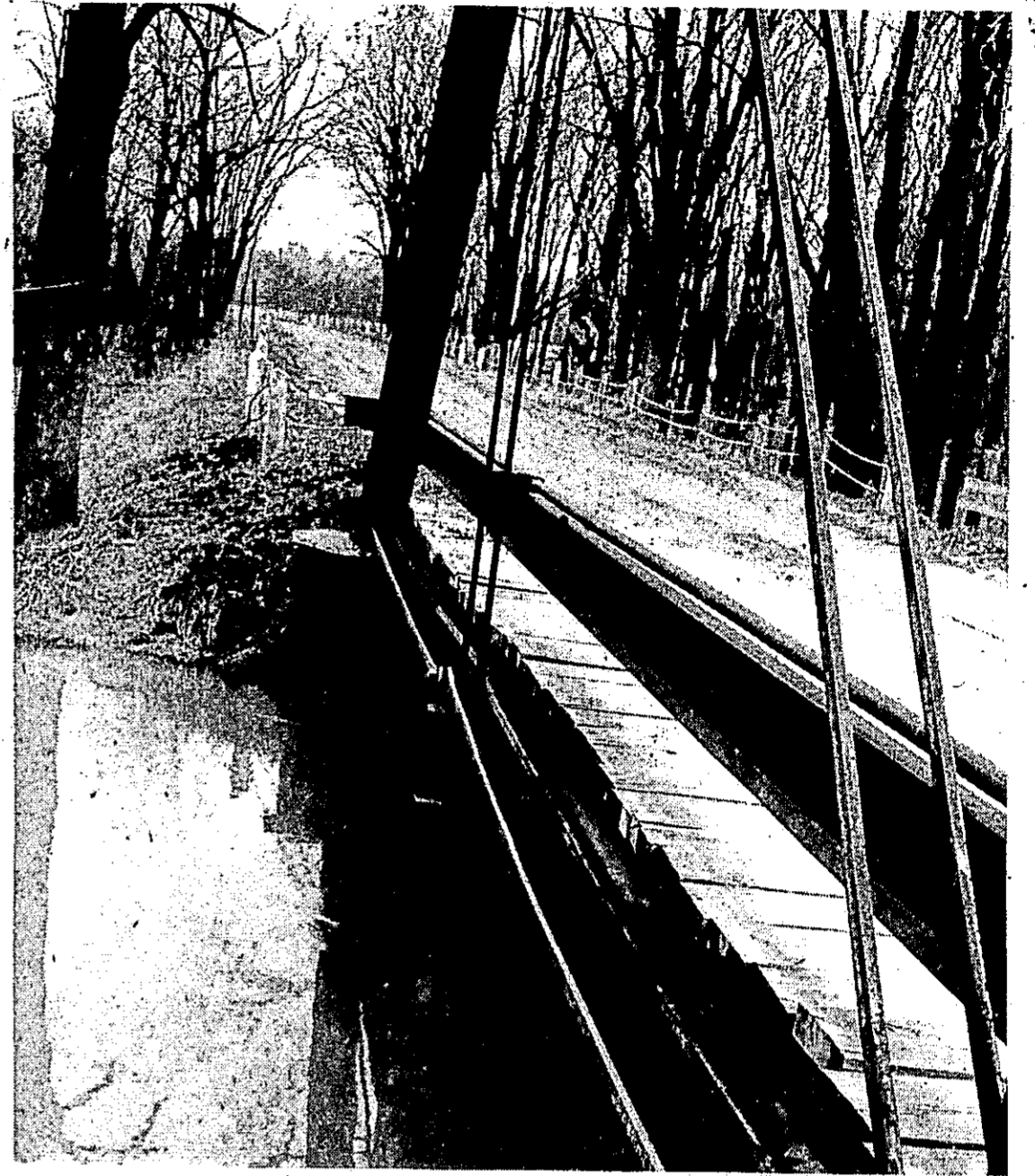
TALLMAN ROAD CROSSING MAPLE RIVER.
