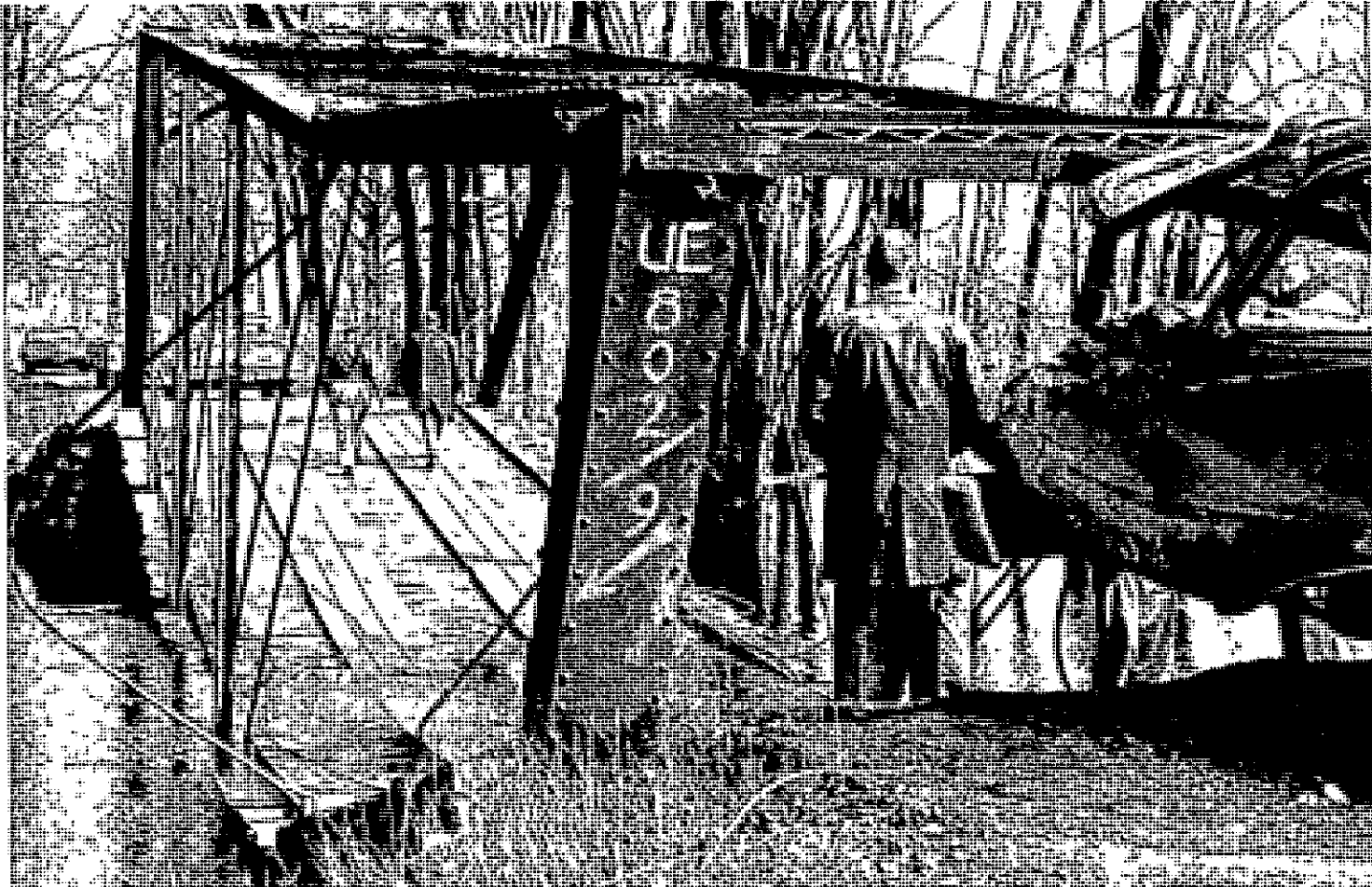
Law officer Hilary Hafner (at left crossing bridge), insurance men and Clinton County Road Commission officials examine the Krepps Road bridge over the Looking Glass River last Wednesday morning after the car at right hit one of the trusses of the bridge and it collapsed. The center of the bridge is resting on the bottom of the river as about two inches of water flows over the top of it.
