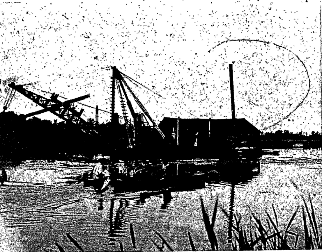
DREDGE AT WORK ON THE MAPLE RIVER
