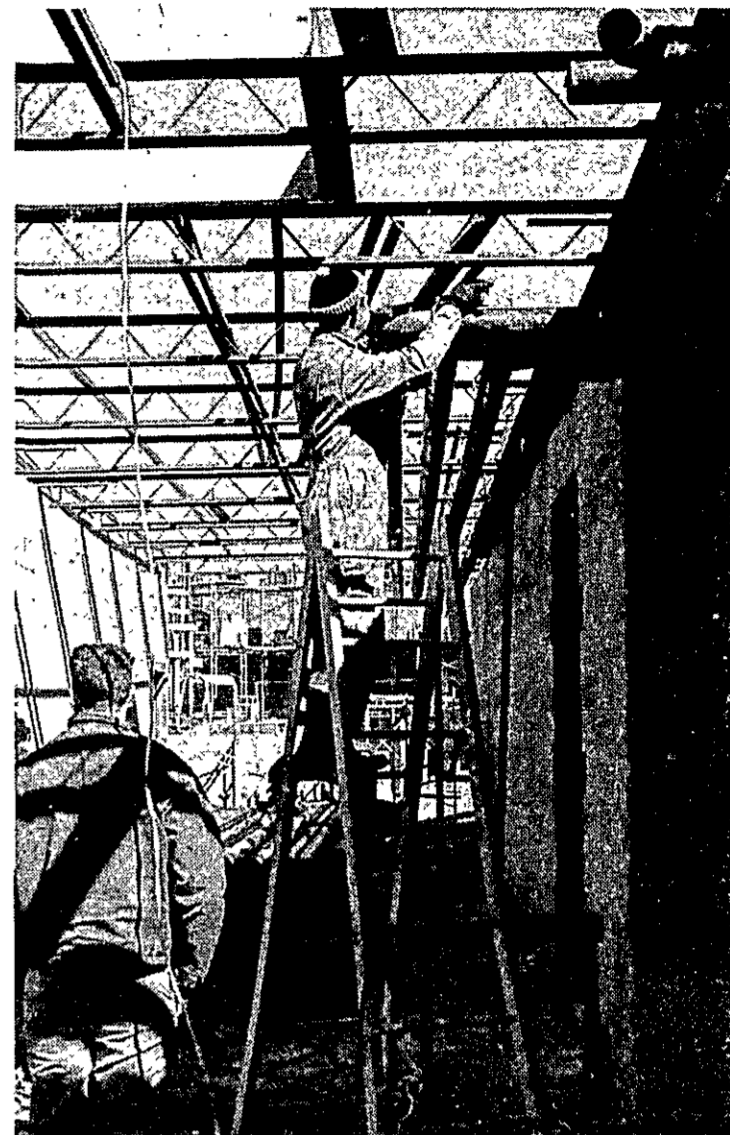
Welders level up piping from the boiler room out into the corridor between the new high school gym (left side of picture) and the electronics classroom (right side of picture at doorway).
