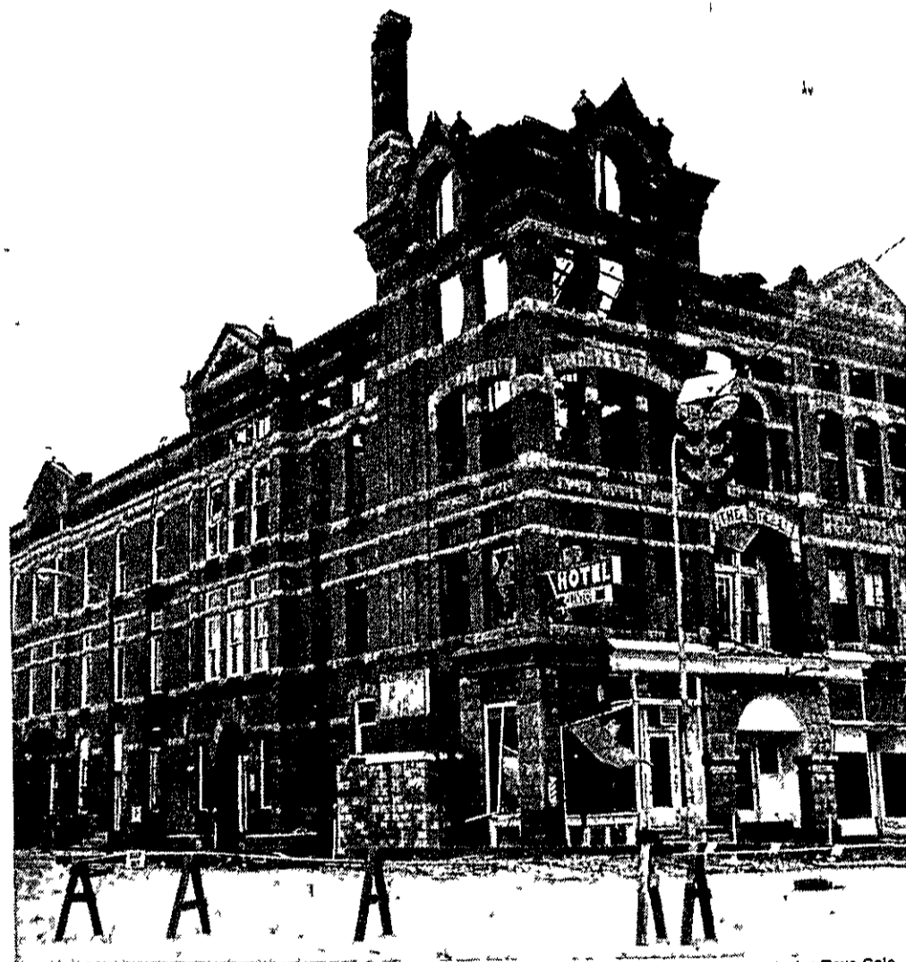
A bleak scene the morning after
