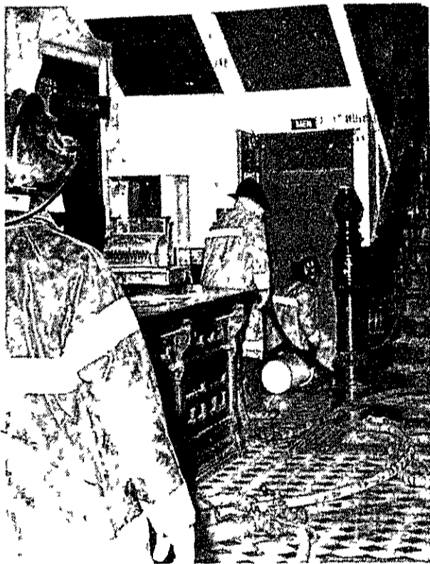
Firemen fight fire spreading from basement
