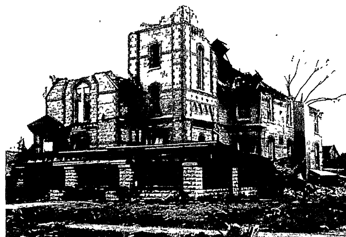
County News Publisher Ron Huard crawled from these ruins of the Charles City, Iowa, Elks Club after a tornado devastated it last May. As can be seen through the windows, the roof and floors collapsed into the building, and a wing of the lodge (not shown in this picture) was completely leveled. Huard escaped injury.
