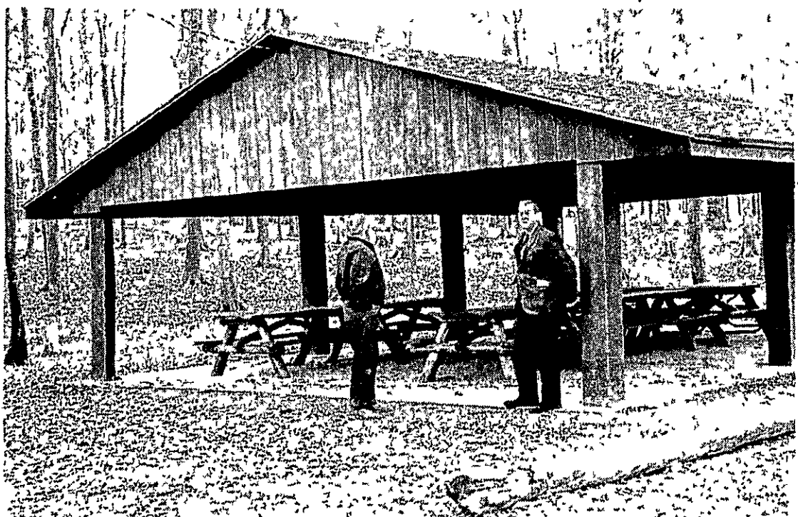
One of the newer structures in the city park is this shelter erected by members of the St. Johns Rotary Club. Park Director Charles Langlois, left, and Park Board President Kurt Becker are shown examining the building to determine extent of necessary repairs.
