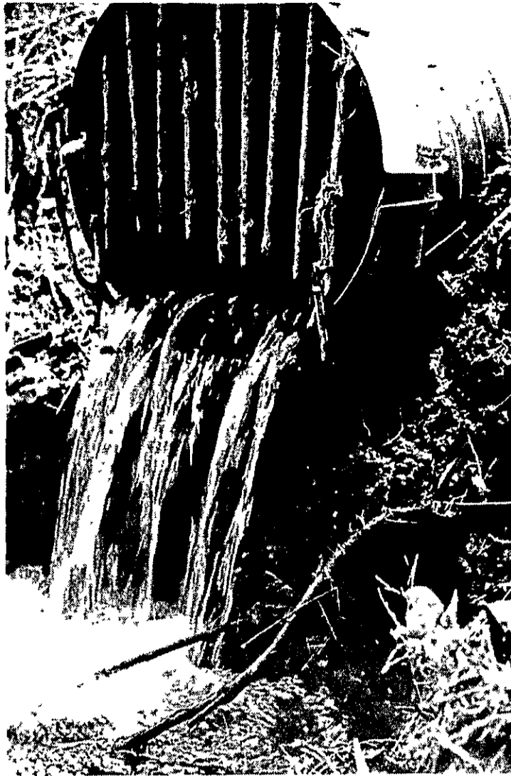
Tile Outlets Should Be Kept Clear
