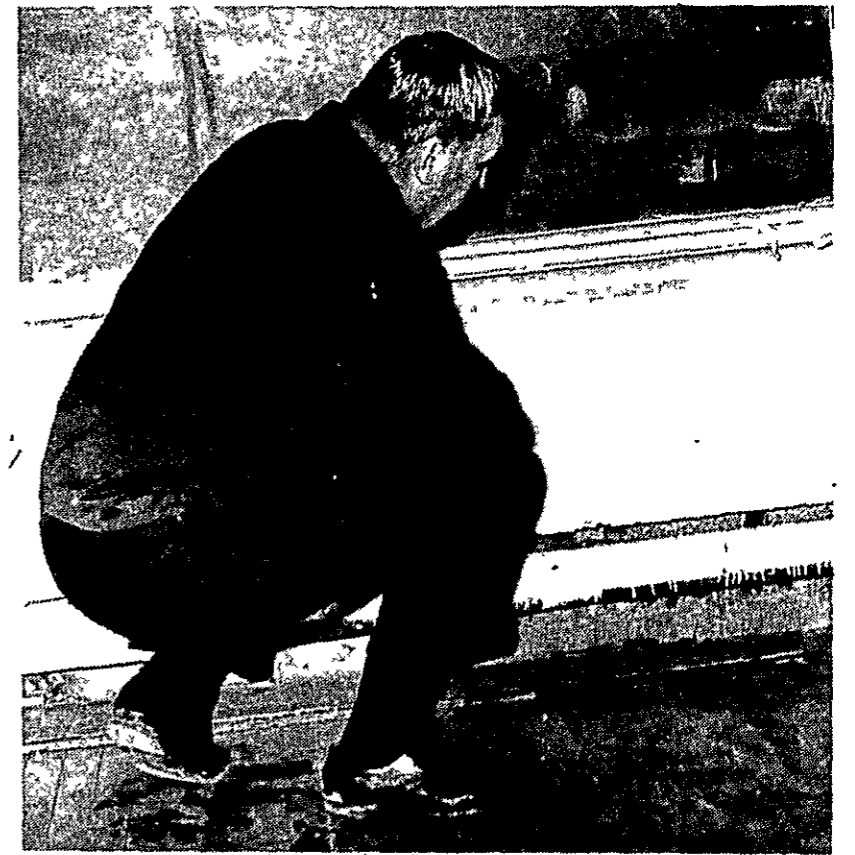
SUPT ROGER CARLSON INSPECTS A COLLAPSED FLOOR
